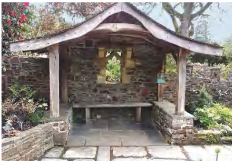
A bower with a 'cruck' roof at RHS Rosemoor, Devon
